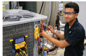
Heating, Ventilation, Air-Conditioning / Refrigeration Approx. 12 mos. | $5,750 🎓
